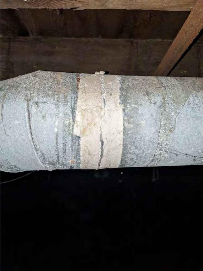
Figure 3: White Duct Tape on vents in basement.
