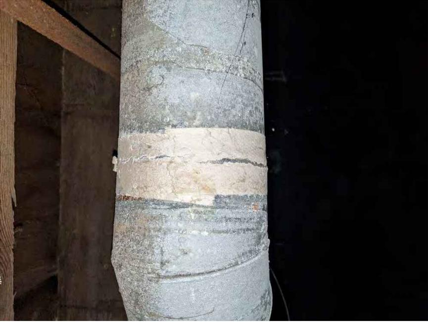
Figure 3: White Duct Tape on vents in basement.
