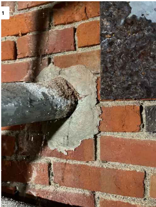
Asbestos Containing Refractory Cement in Basement
