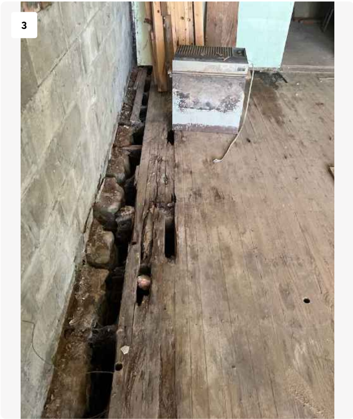
Structural Deterioration on First Floor, West Side of the Building
