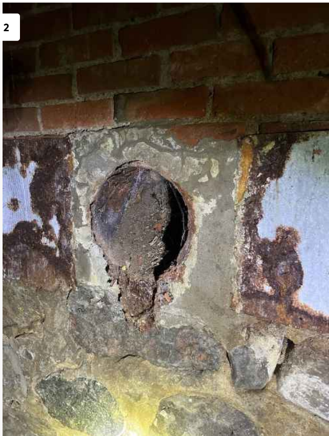
Asbestos Containing Refractory Cement in Basement
