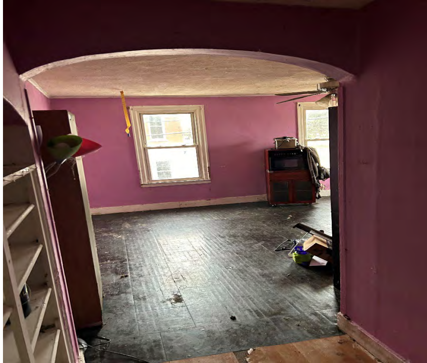
17. Upstairs bedroom of subject building.
