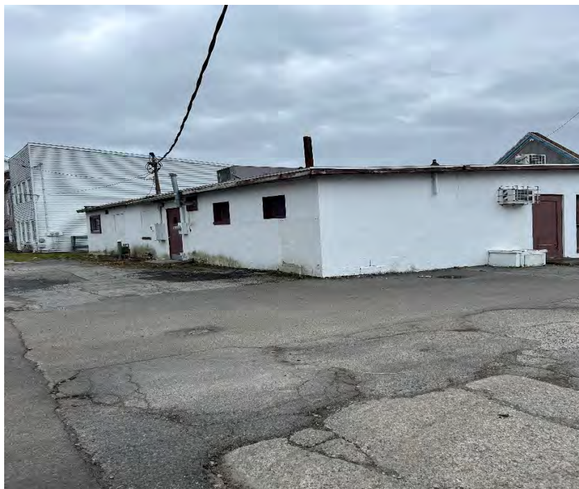
6. View of adjacent East building to subject property.
