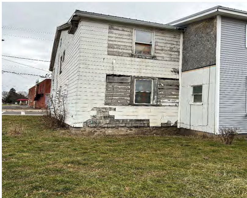
2. Eastern exterior of the subject property.
