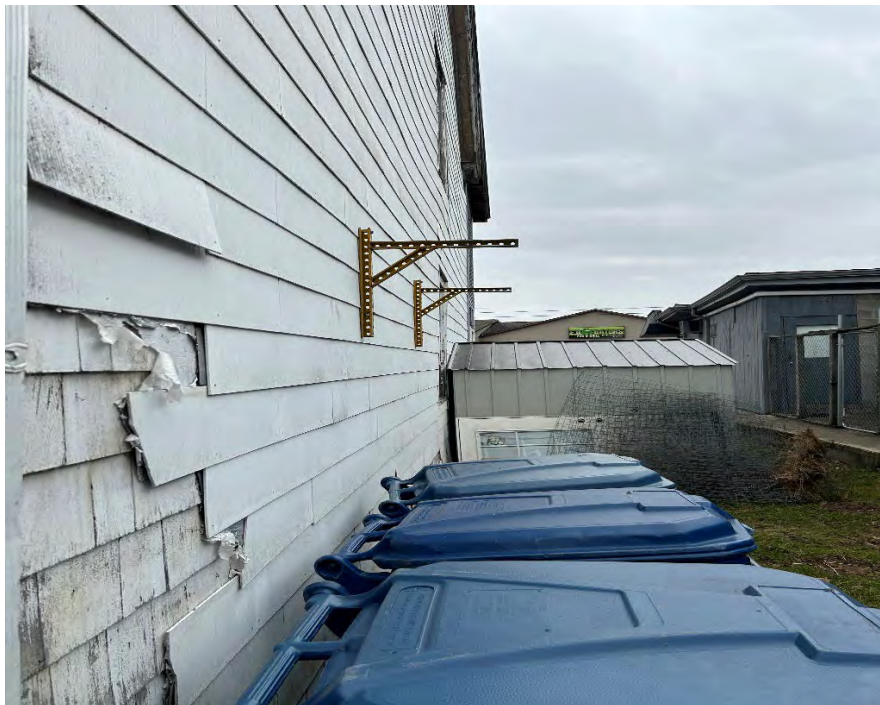
4. View of West side of subject building.
