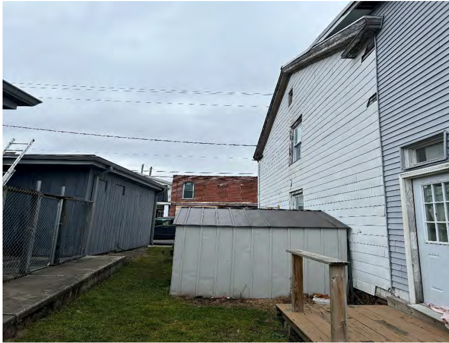
3. Northwest exterior of subject building.
