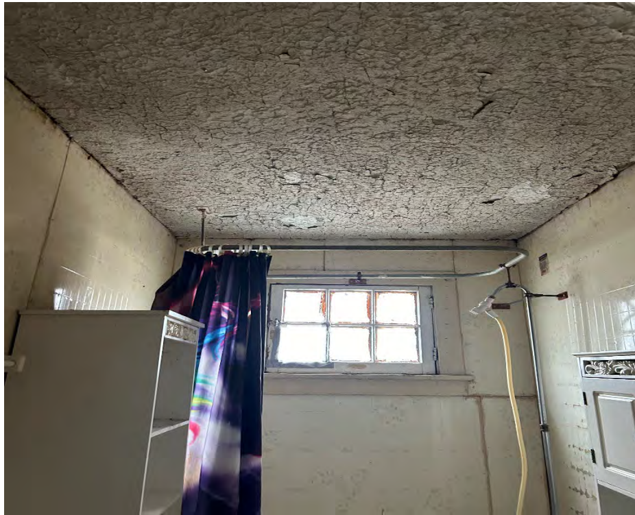
7. View of upstairs bathroom ceiling.
