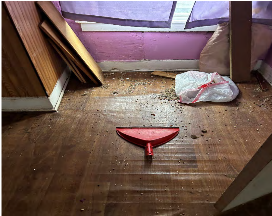
19. Rear upstairs bedroom with debris.
