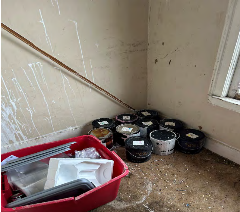
13. Paint cans in upstairs bedroom of subject building.
