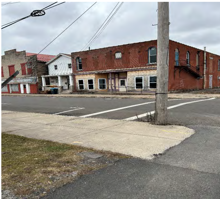
5. View of surrounding properties directly across Canal Street.
