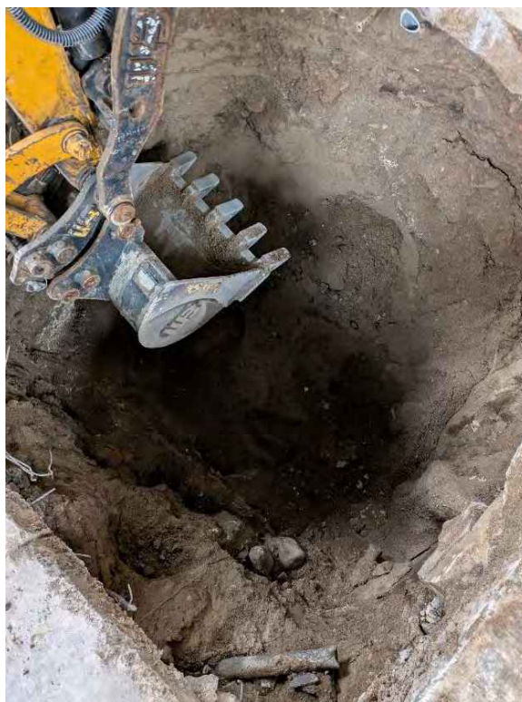
8. Excavation at south lift. Brick fragments and hydraulic system piping shown.
