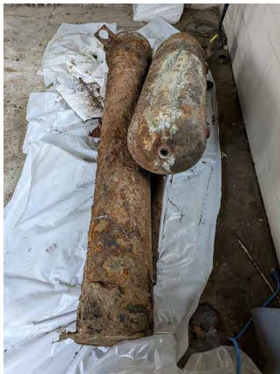
7. Removed south lift and hydraulic oil tank staged on poly sheeting.
